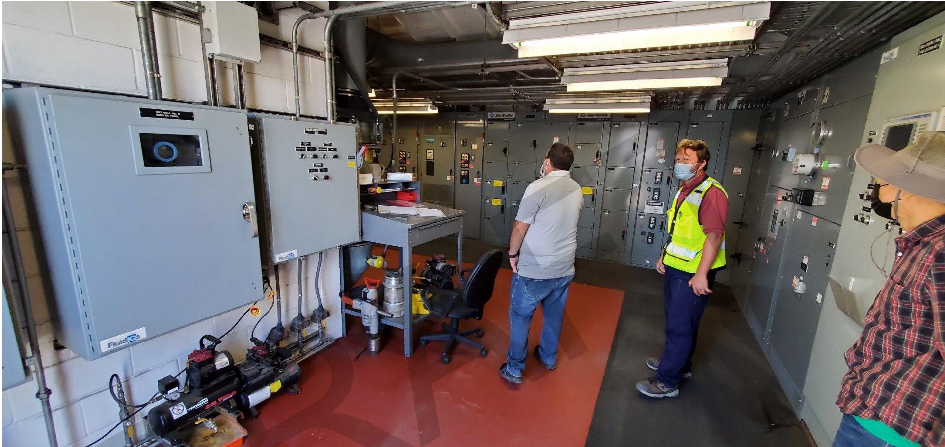
A6. Example of electrical systems inside a building in the WQCP area.
