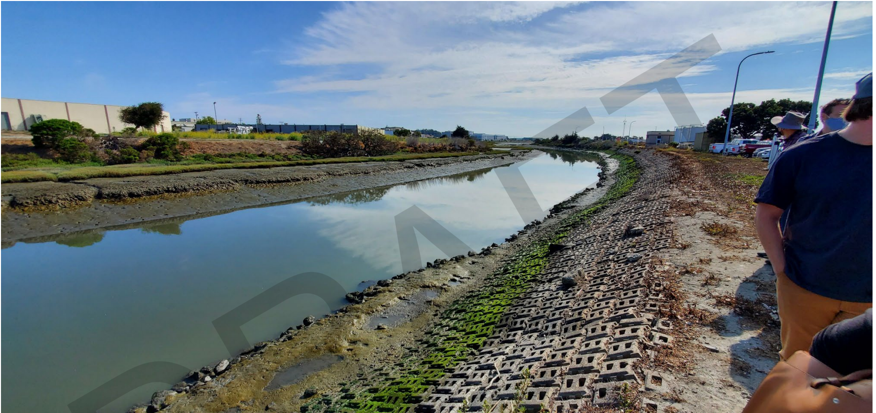
A1. View of Colma creek channel looking downstream from the south (WQCP) side.
