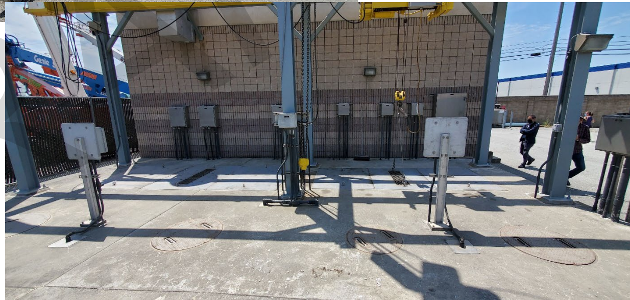
A8. Equipment at Pump Station 4.
